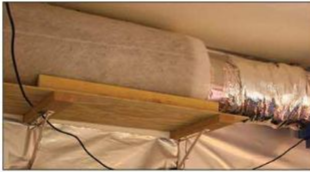
An air filter sits high in the room to capture hot spent air where it gathers.
